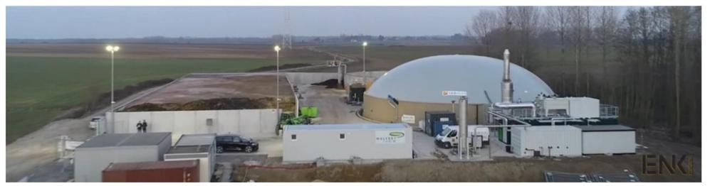
1 ton of manure + corn silage (max 20%) + green organic waste  $\rightarrow$  900 kg liquid digestate 6 UN (mostly available) + 5000 MWh
