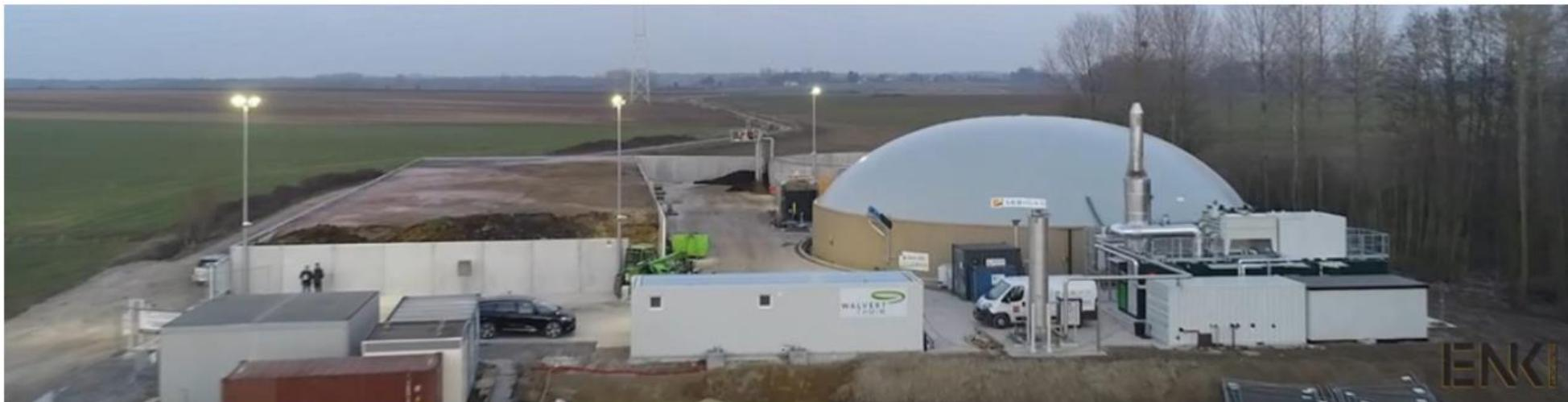
1 ton of manure + corn silage (max 20%) + green organic waste → 900 kg liquid digestate 6 UN (mostly available) + 5000 MWh
